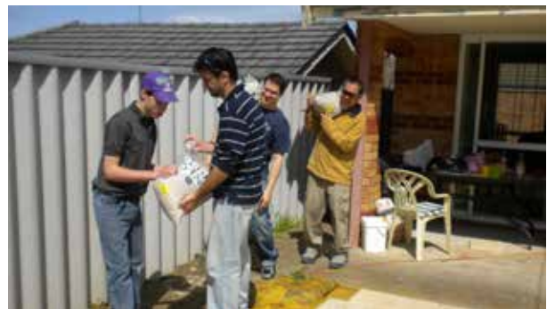
Team paving effort at Cam & Tupea's house.
